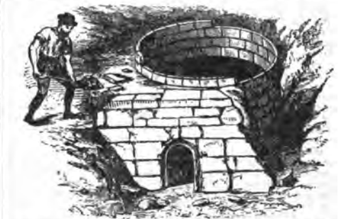
FIG. 4.—Roman kiln found at Castor. The low arch is for the insertion of the fuel; the pots rested on the perforated floor, made of clay slabs; the top of the kiln is missing,—it was probably a dome.
